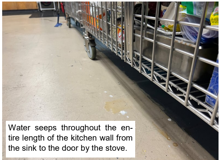
Rainwater also comes through the paint and runs down the wall in the kitchen as well as through the wall and out from under the wallboard.
