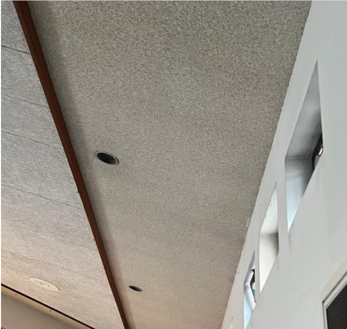
This area of ceiling shown above continues to drip onto the pews near the heater intake during rains.
